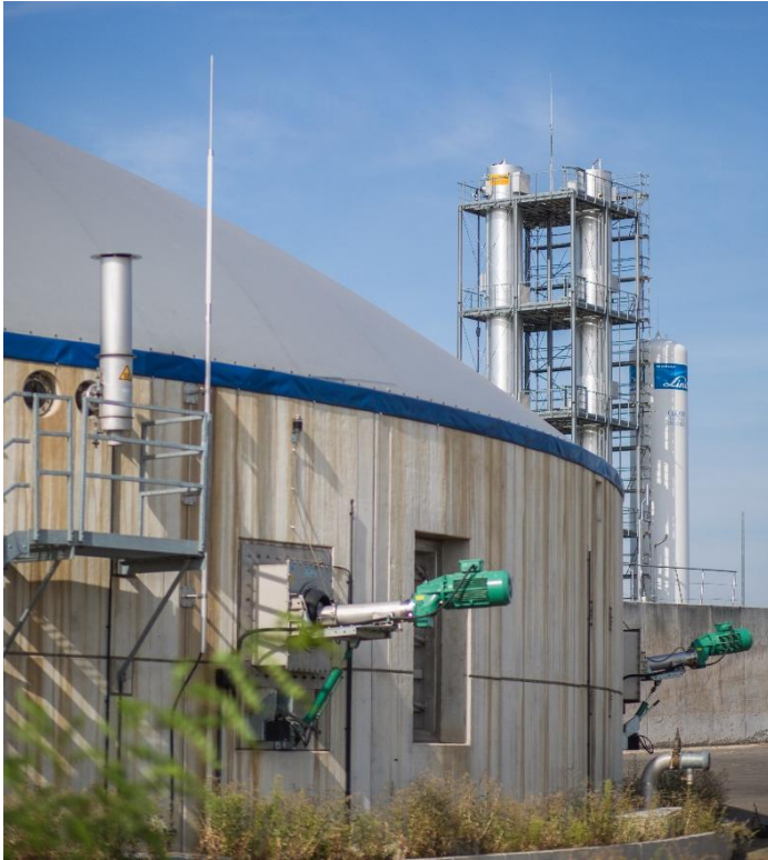
Fig. 1: Biogas plant (foreground) and trickle-bed reactors for biological methanation at Pirmasens-Winzeln Energy Park
