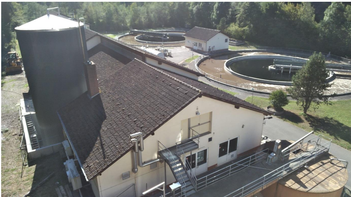
Fig. 1: Photo of the machine hall of the Felsalbe sewage treatment plant with new high-performance digestion system (on left). Two sedimentation tanks can be seen in the background.
